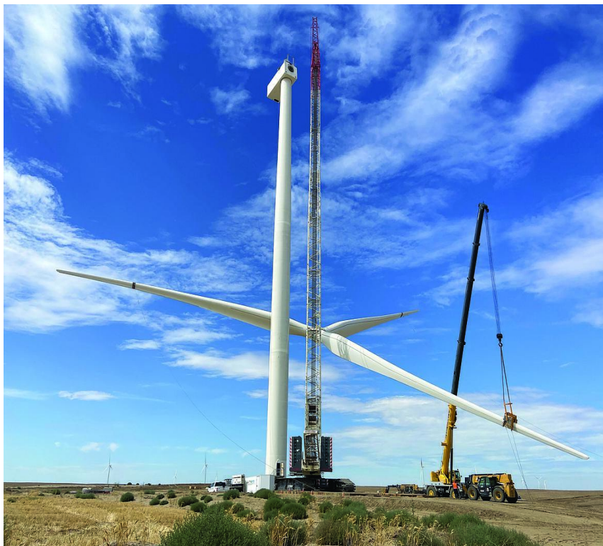
1 Construction of the Rattlesnake Flats Wind Energy Project
