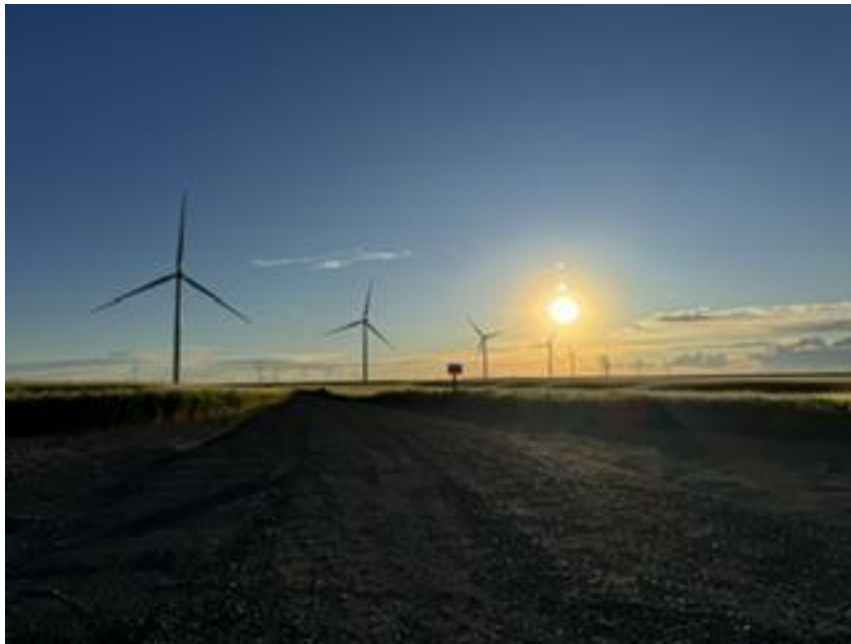
3 Completed wind turbines at the Rattlesnake Flats Wind Energy Project
