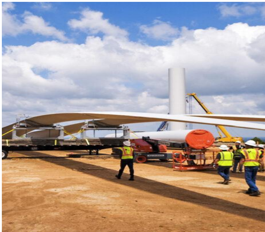
2 Transportation and installation of wind turbine components during construction.
